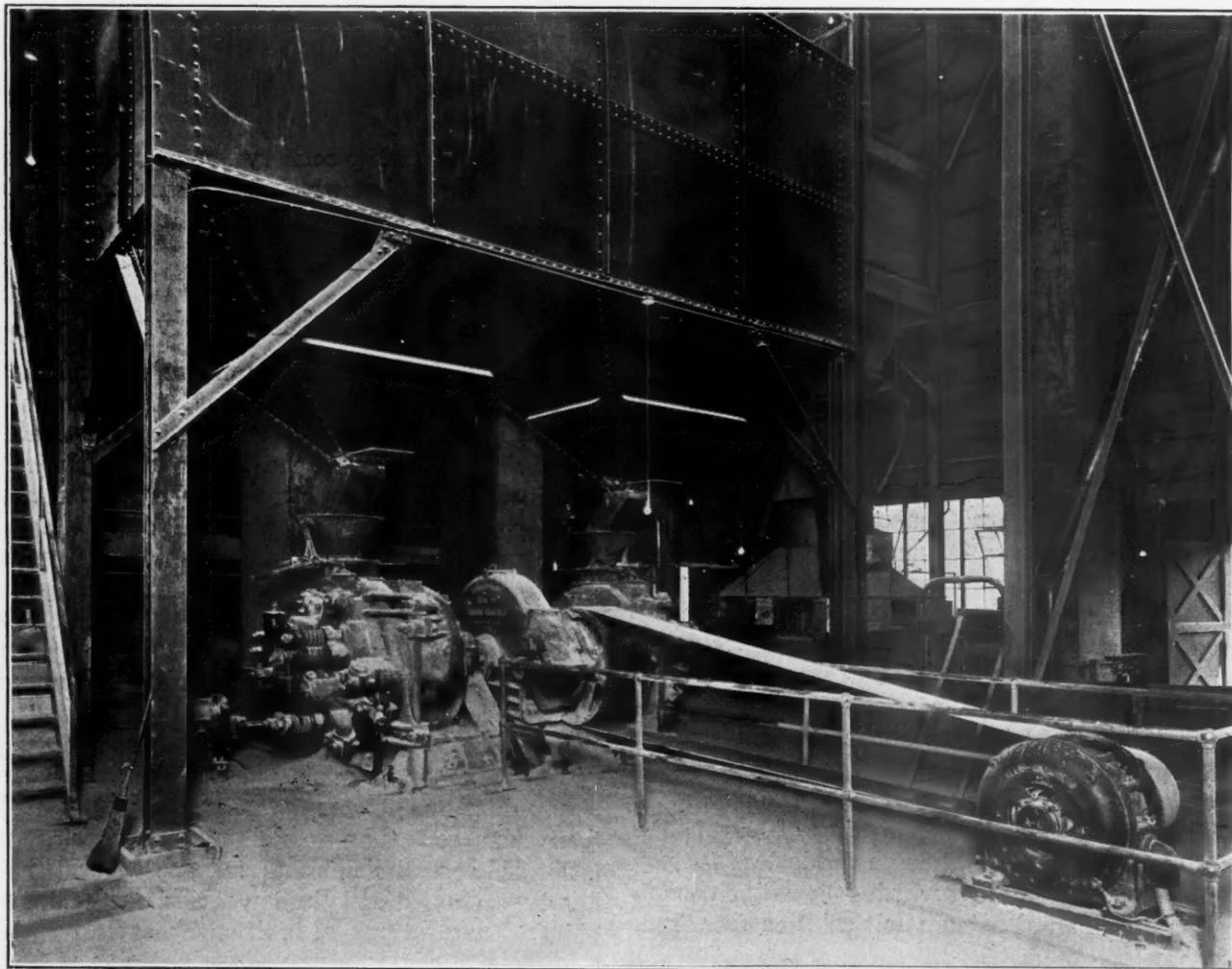
Close Up of One of the Large Preliminary Grinding Units. With Material Proportioning Machine in the Right Background.
